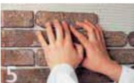
Then apply the strip in a sliding motion. Always start with the corners or wall edge and mix strips from different boxes
