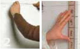
Establish the height of the area to be covered. Then establish the average height of a brick slip, by stacking 10, measuring and dividing by 10. You can then estimate how many brick slips are required to cover the wall. Remember to allow for the joints, ideally 10mm, though this may need to be flexible depending on the wall and brick slips sizings you have established.
