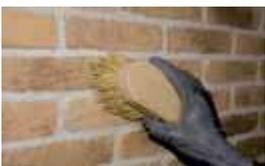
Clean away the extra mortar with a stiff dry brush before it has completely dried.
