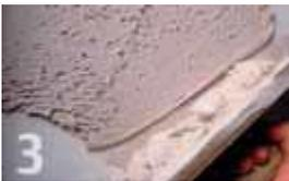
Apply the adhesive in sections of  $\frac{1}{2}$  m<sup>2</sup> so that it doesn't dry before you fix the brick slips and so that stains from spotting and spilling can then still be easily removed. It's important to source a flexible adhesive that is suitable for the surface you plan to fit the brick slips to. (i.e concrete, wood, metal). It's also vital to follow the manufacturer's instruction of use
