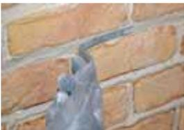
When the joint begin to harden, tighten it with a narrow trowel or coursing tool. Do not touch the joints as they are fresh and they have not sufficiently cured.
