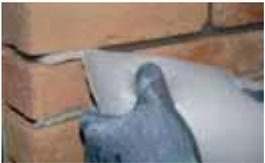
For best results we recommend the use of mortar. Use a mortar plastic bag or a mortar gun. Test the texture and colour on a small section of the fitted slips to ensure you have the right concentration and colour. It's important to use the same proportion of water, to avoid colour variations, once started.
