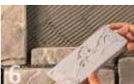
We also recommend that you apply the adhesive on the back of the slips as well as the wall-surface.
